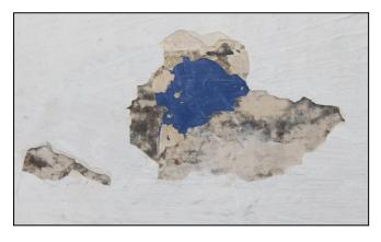
flaking off on all of the walls. In the trial area in places the oil bound paint layer has attached itself to some of the original red and blue paint and cannot be separated by mechanical or chemical methods without destroying the original decoration. This is why patches of this paint remain in the trial area. The paint began life as a cream colour, but has discoloured to a grey/ brown tone; it is very smooth on the surface.
