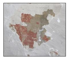
"I started on the south west end of the south aisle (near the font), in between the wood panelling and the window above. The top coat, the most recent is a neat white lime wash applied with course brushes as the brush marks are quite evident. Over time this white lime wash has discoloured to a grey hue. In many places the lime wash has become detached from the coat of paint beneath. The layer beneath
